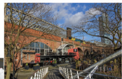
Below: Having been disused for many years, the condition of the Cornbrook and Great Northern Railway Station was revived when a route for the Abrahams branch of the Metrolink was sought. The Cornbrook Viaduct was found to be in better condition and was refurbished 1990-91. The line to Abrahams opened the following year.
